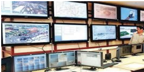
Fig 2.2: Bangalore Traffic control Room.
