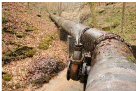
Figure 1: A Trivial Water leakage Location
